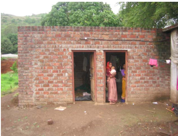
Fig. 1 The refrigeration rooms
