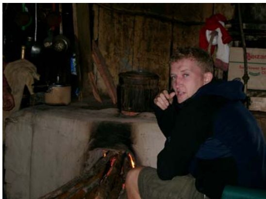
Figure 1 – An example of the type of stoves in use in the Sagarmatha region of Nepal. Note the carbon build-up on front of the stove.
